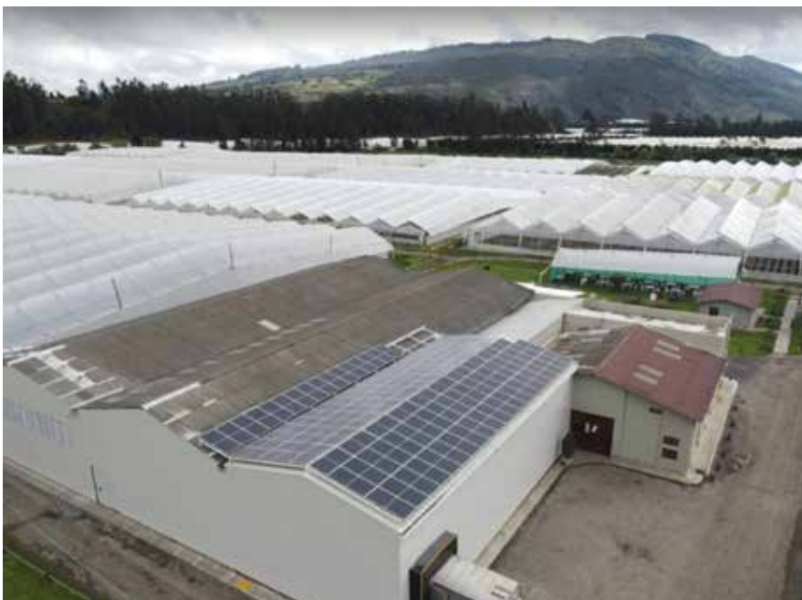
CONSERVING ENERGY Two of the postharvest buildings at Ayura Eclipse Pride Flowers in Colombia are equipped with solar panels, which provide about 60 percent of the farm's energy.
